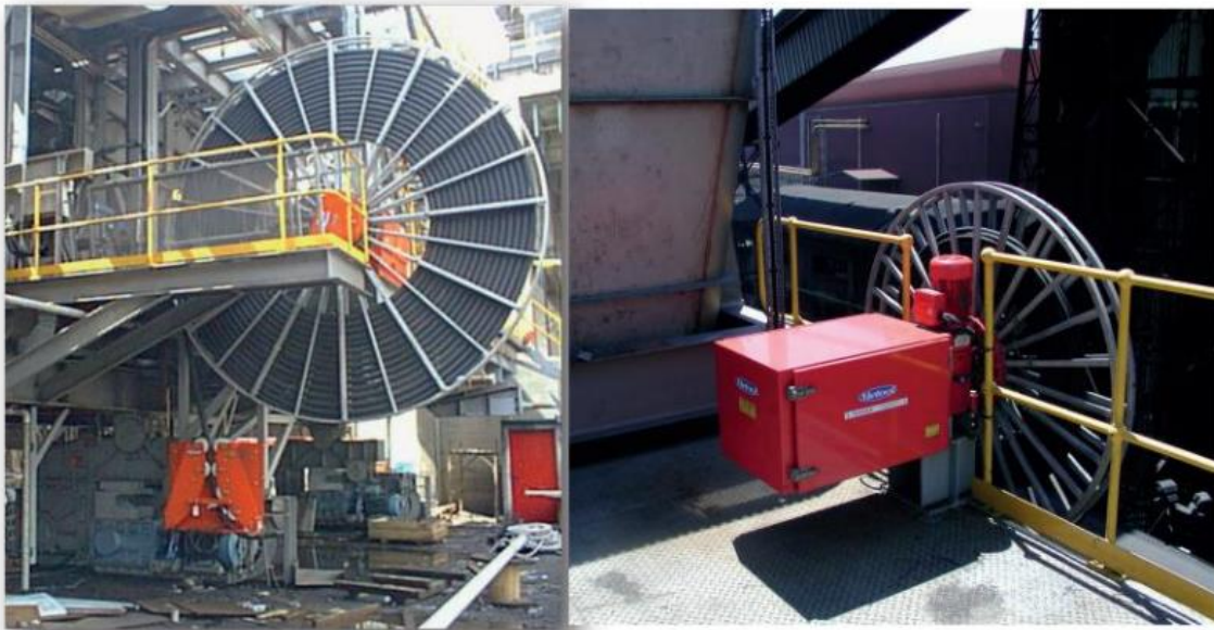
Power & Fibre Optic Cable Reel installations on Coke Oven Machines
